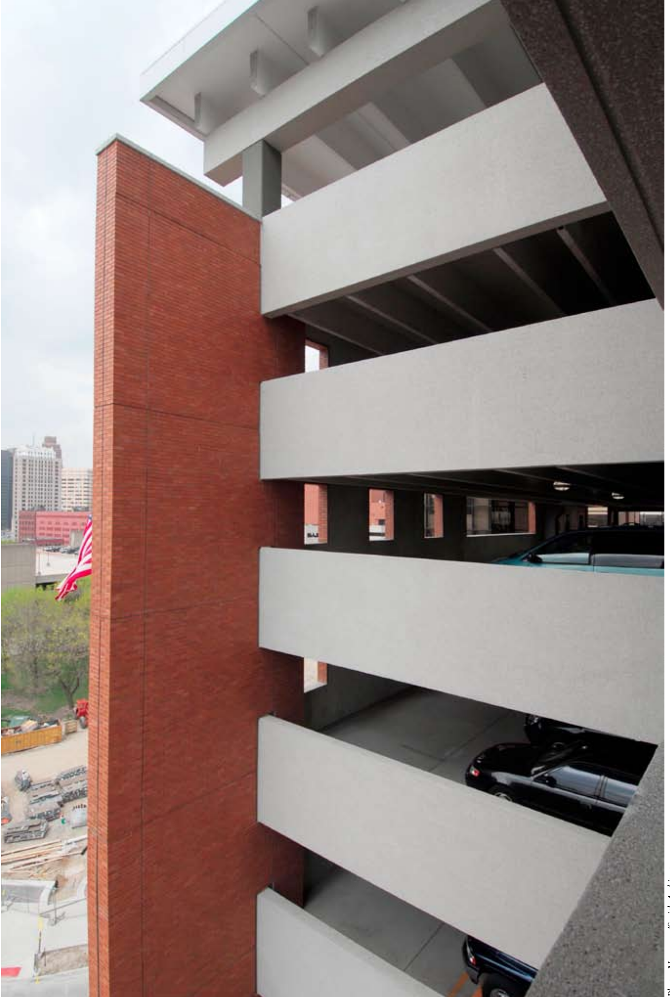
Photo: Neumann/Smith Architecture
