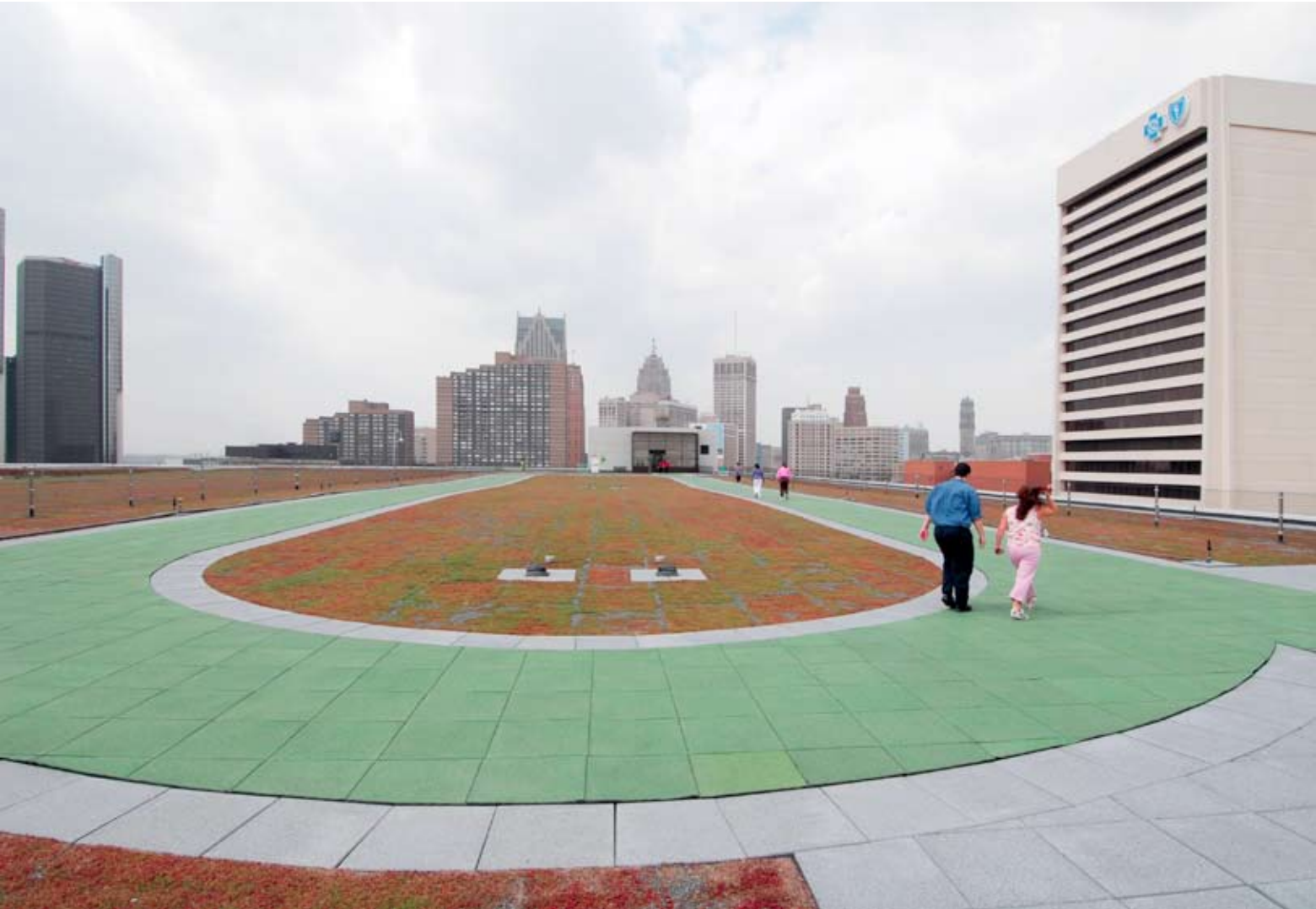
The roof of the Blue Cross/Blue Shield parking structure features a 1/10th-mi walking track and planted vegetation. Photos: Neumann/Smith Architecture
