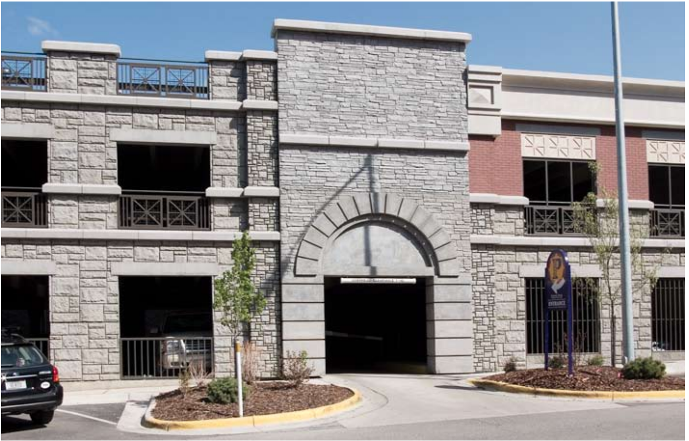
Two colors, three textures and inset brick produced a look for the Jackson Street parking structure that helped it fit into its neighborhood. Photos: Cullen Architecture & Design.
