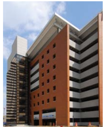
The Blue Cross/Blue Shield facility in Detroit is one of the first LEED-certified parking structures.
