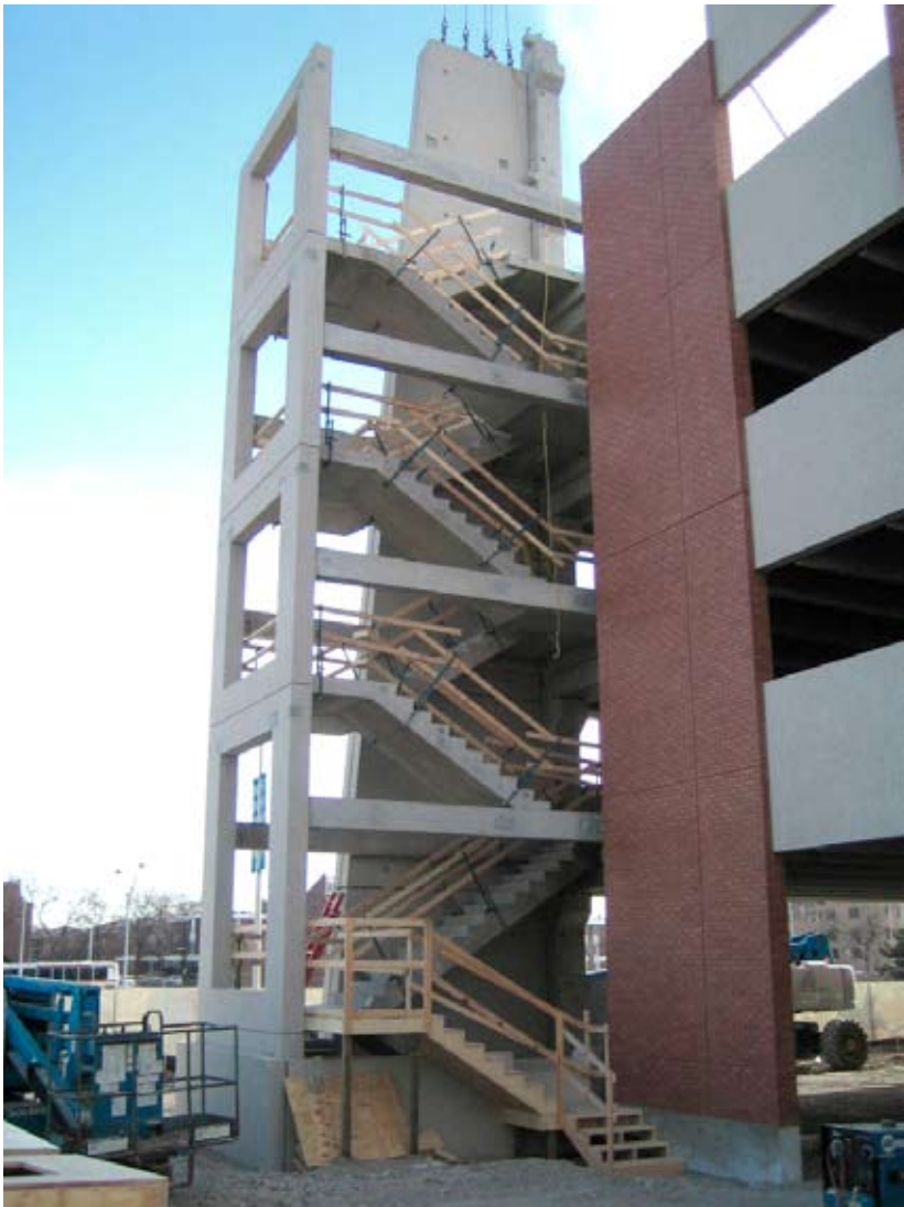
Photo: Neumann/Smith Architecture
